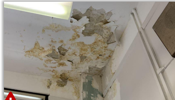
Failed plaster/interior finishes
