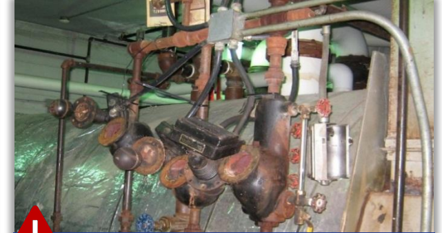
Corroding distribution piping
