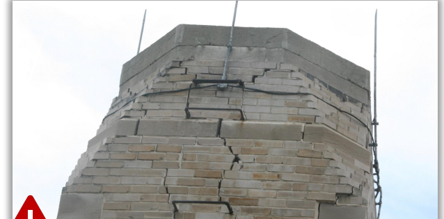
Displaced Chimney Masonry
