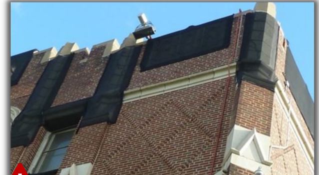
Temporary stabilization of brick erosion
