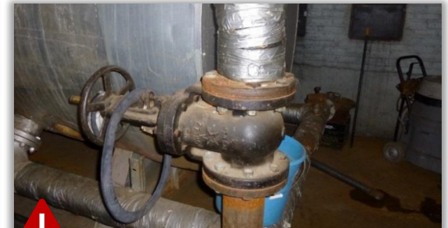
Failing heat distribution piping
