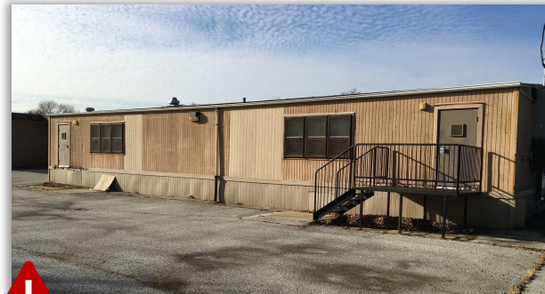
Existing modular building
