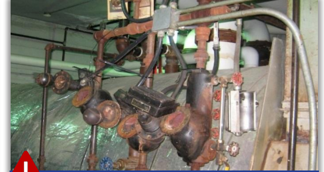
Corroding distribution piping
