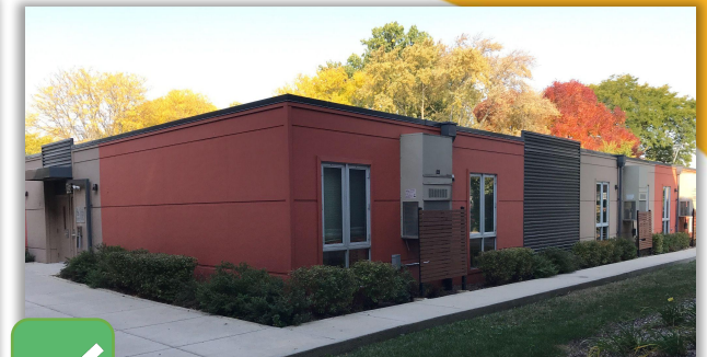
Replacement modular building
