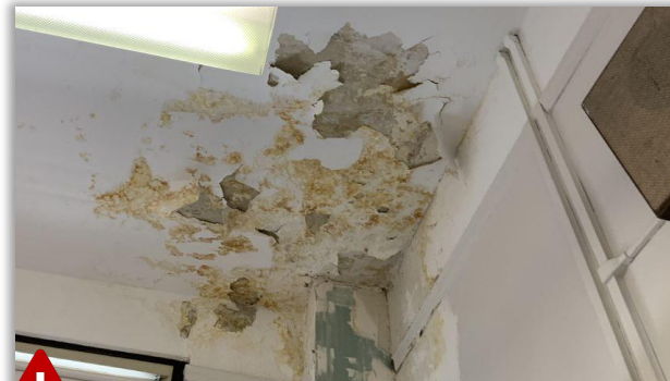
Failed plaster/interior finishes
