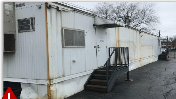
Existing modular building
