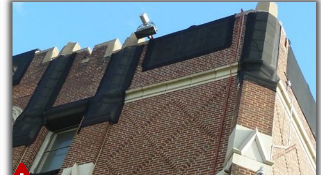
Temporary stabilization of brick erosion
